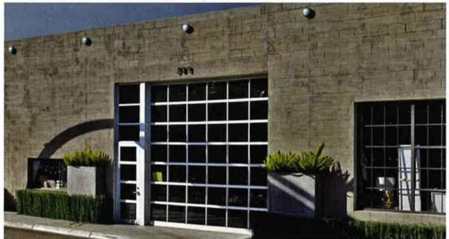
Shot blasted precision concrete block
