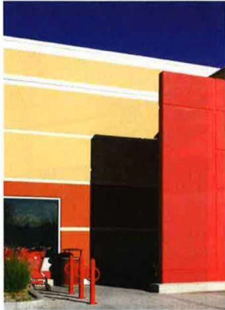
Painted tilt up concrete panels
