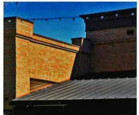
Brick walls with standing seam metal roof
