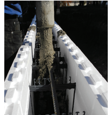
Concrete Placement
