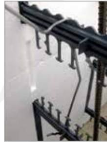
Vertical Clips in Place
