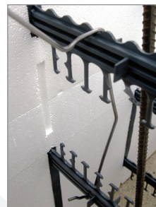
Vertical Clips in Place
